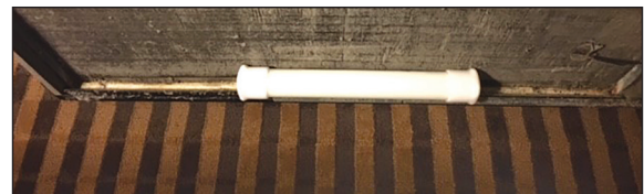
OPTION 2 FOR PTAC INSTALL: Place MiniFresh in return air at base of evaporator.
